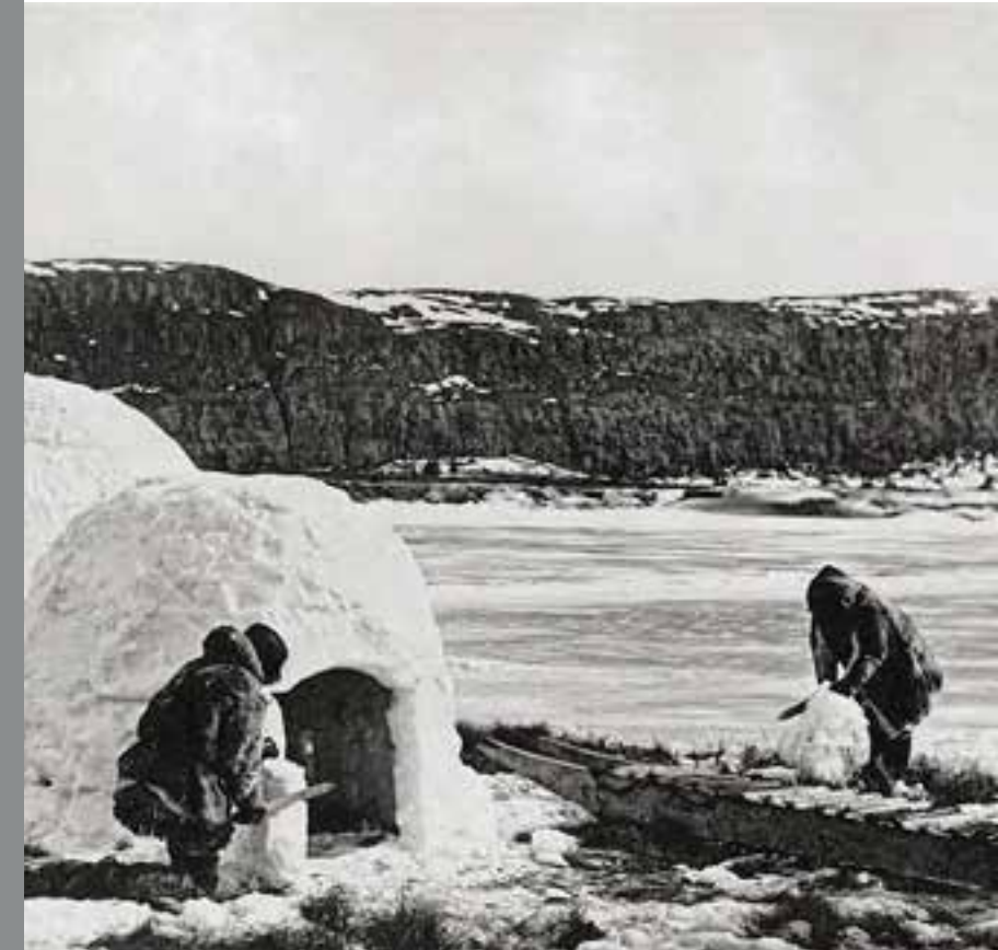
Building a snow house at Little Whale River, Que., in 1872. This house is representative of those Inuit build throughout the Nunavik region each winter.
