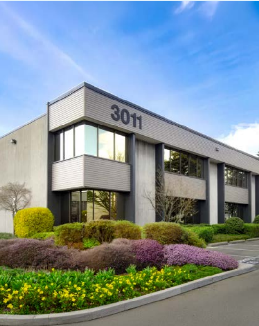
KNIGHTSBRIDGE OFFICE, RICHMOND, BC Dual-Fuel Rooftop Heating & Cooling System Replacement
