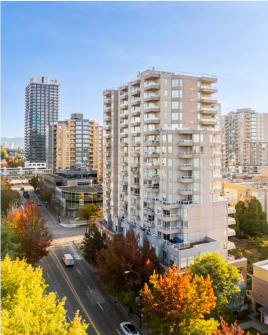
WESSEX GATE, VANCOUVER, BC Hot Water System Retrofit
