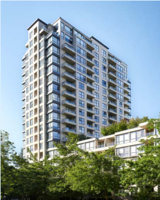
THE REMINGTON, VANCOUVER, BC Dual-Fuel Fresh Air & Heating System Retrofit
