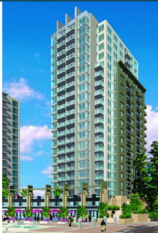
Now under construction – and virtually sold out – is Astoria, Concert’s first residential project in Victoria.
