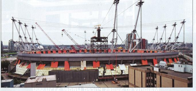
"an architectural signature" for the city. When the new cable-supported roof is opened, it reveals an area of 100 metres by 85 metres, the same size as the field below.
